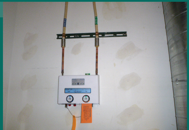
MediTrac® CMT connection to Dental Manifold.
