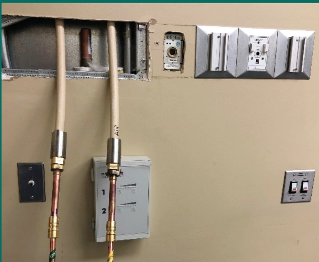
Flameless addition of medical gas outlets
